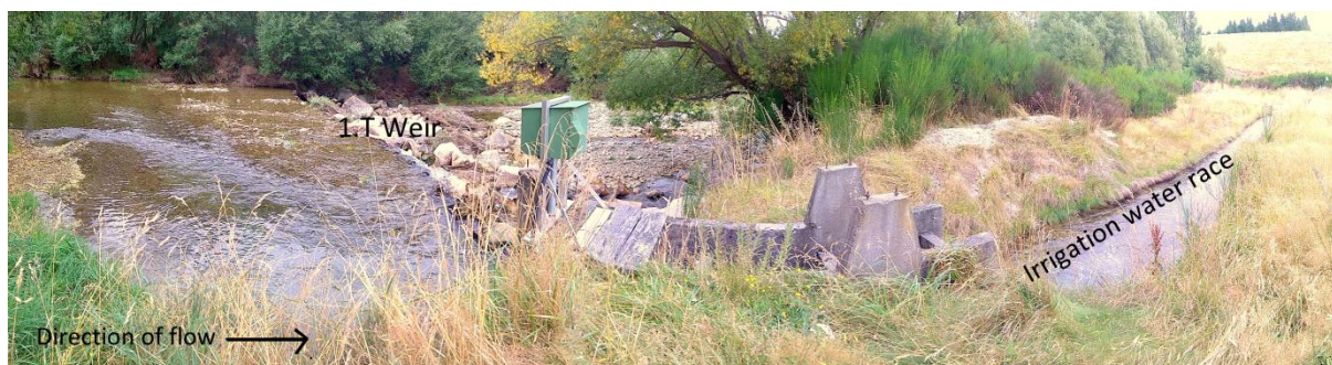
Figure 2.2. A panorama of the water abstraction weir, 1.T clicked during the abstraction and the seasonal low discharge period in March, 2019. Downstream of 1.T, behind the green boxed gauge, the dry tributary bed can be seen while >50% of the discharge runs into the concrete irrigation water race.
