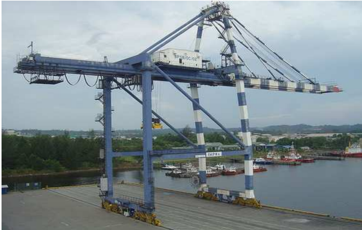
Figure 2.3 An example of quay crane
